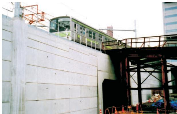
**Figure 24. GRS-RW supporting a rapid transit, near Shinjuku station in Tokyo (Yamanote line): (a) typical cross-section (all dimensions in m); (b) under construction (1995–2000); (c) completed wall**
